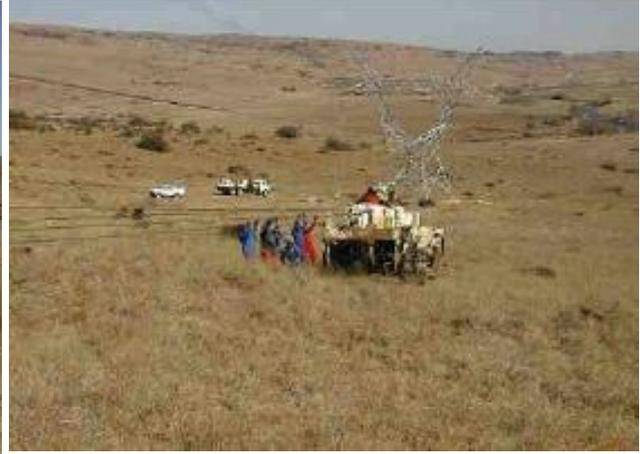
**Stringing pilot cable with pilot tractor**
