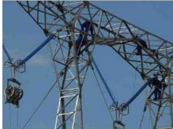
**Using pulleys to hoist cable**
